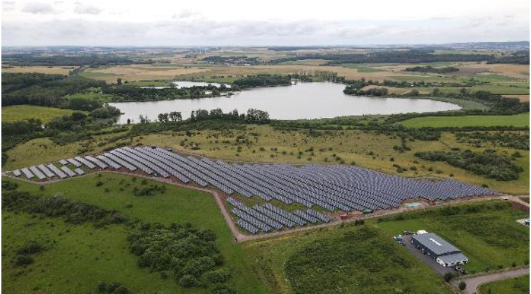
Morhange - 9 MWp - France
