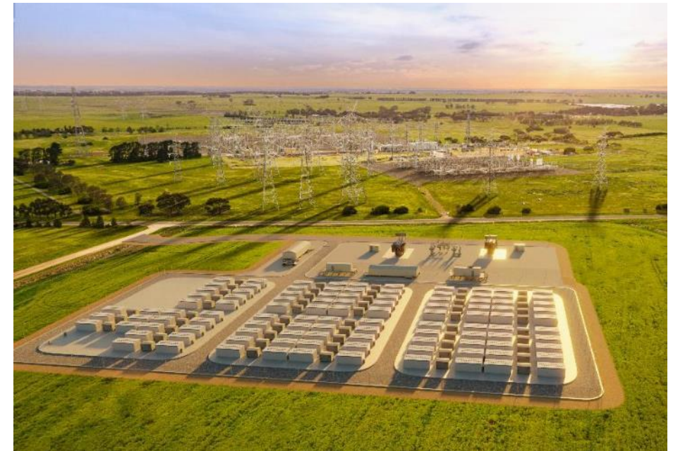
Victorian Big Battery – 300 MW / 450 MWh – Australia
