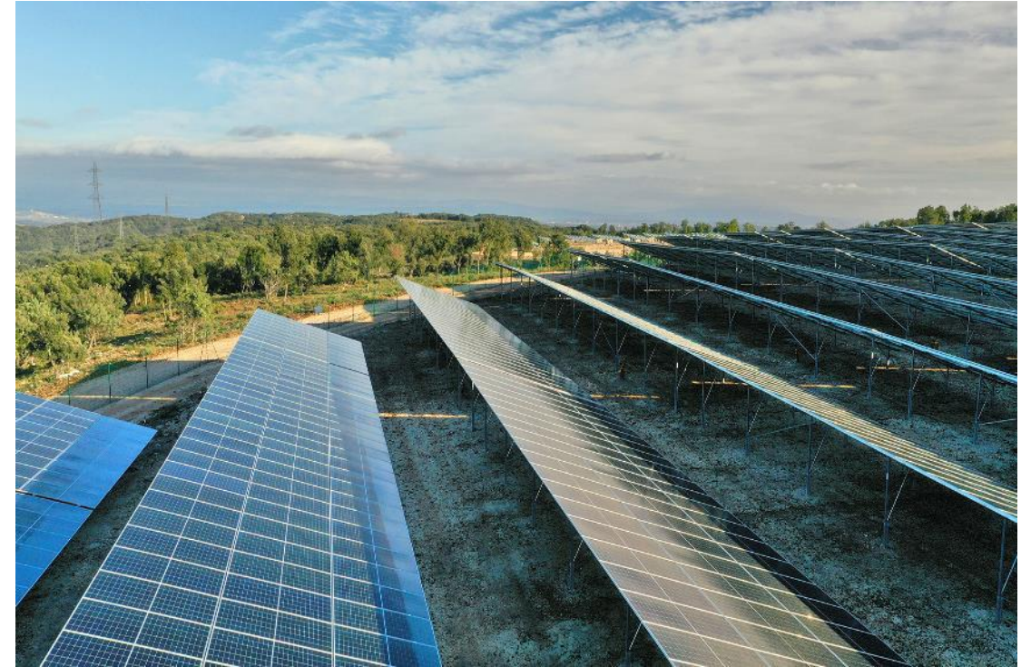
Ecarpière – 14 MWp – France
